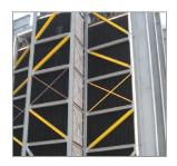
For HRSGs where transport and weight limitations allow, the main steel support structure is integrated and pre-fabricated with the boxes in a design that is the ultimate in constructability.
