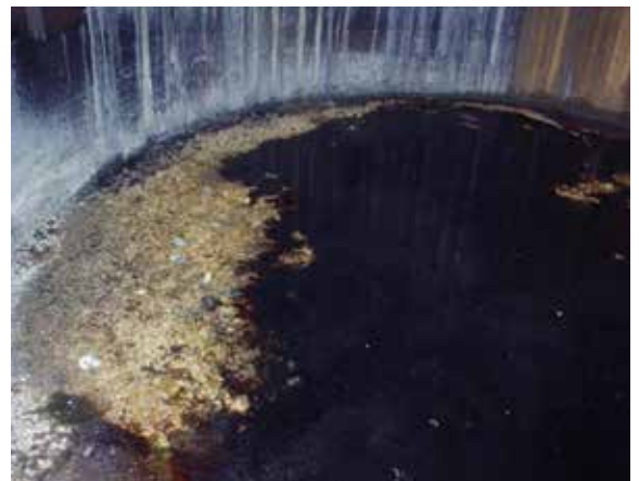
Stack Corrosion Inspection
