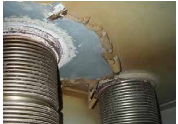
Inspection of External Penetration Hot Spot
